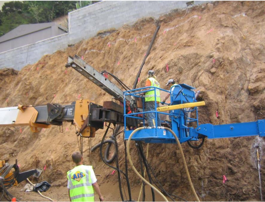
Soil nailing (installation)
