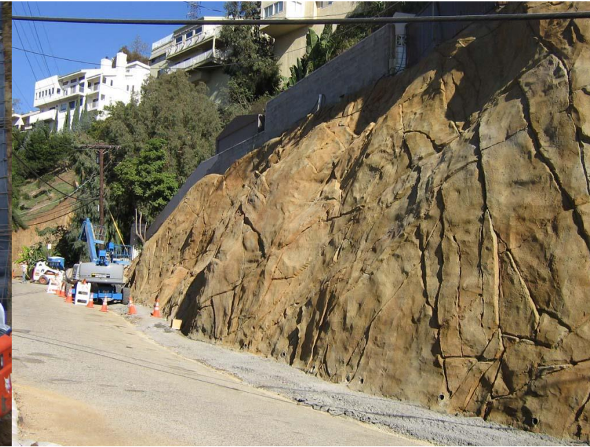
Soil nailing (final)
